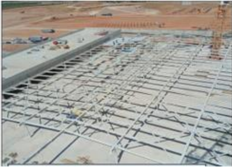
Terminal Building Roof Steel Works
