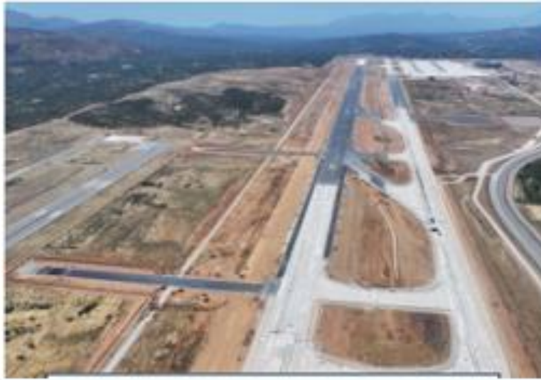
Runway Concreting & Asphalt Works
