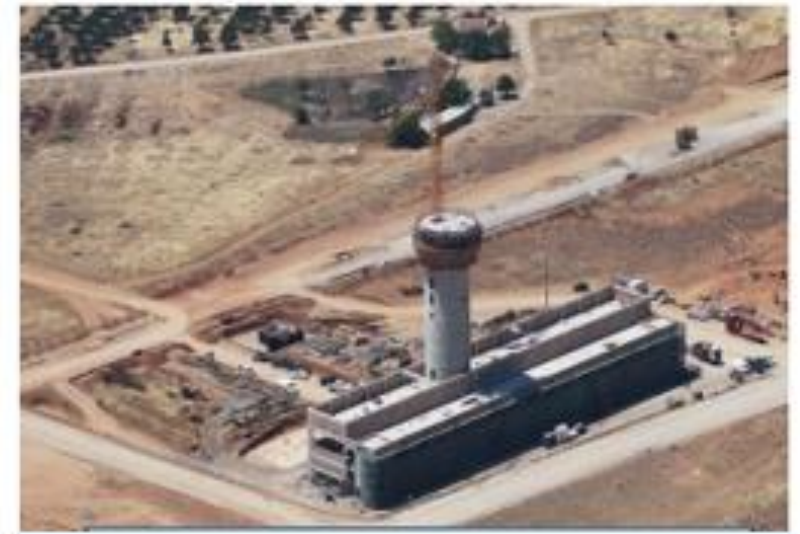
Control Tower Architectural and MEPF Works
